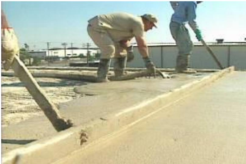
Vermiculite based roof screed being placed
