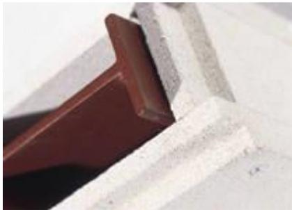
Boards containing vermiculite being used to encase structural steel to provide fire protection
