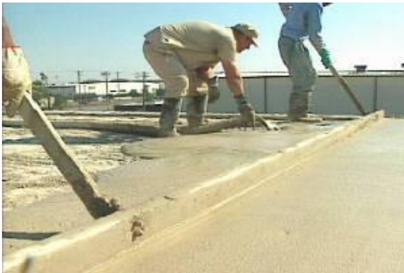
Vermiculite based roof screed being placed
