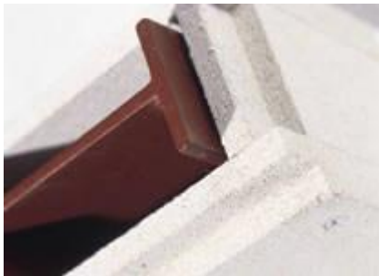
Boards containing vermiculite being used to encase structural steel to provide fire protection
